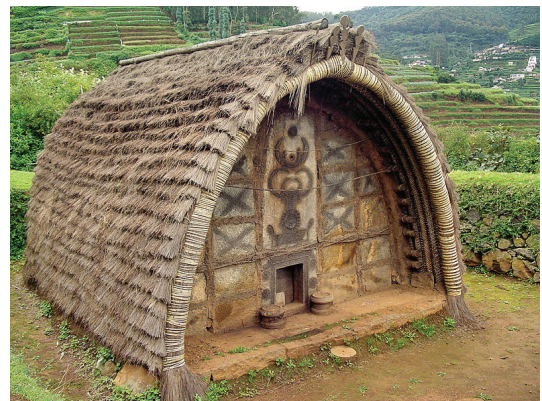
The Todas traditionally live in small villages called munds. Their huts are built of bamboo and are then thatched. The front and back of the hut are usually made of stones. The hut has a tiny entrance—about 3 feet by 3 feet—as a means of protection from wild animals. The front of the hut is decorated with a kind of rock mural painting.
